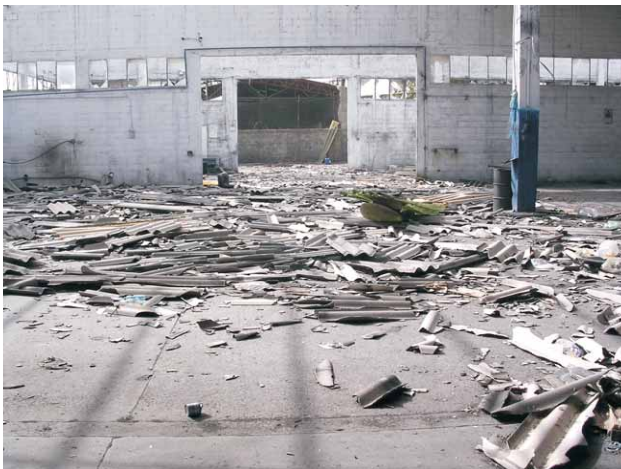
The removal and disposal of rubble remains a major activity to be undertaken prior to resettlement, issues associated with asbestos need to be handled carefully so as not to expose workers to unnecessary harm
