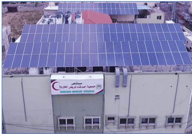
Figure 13: Existing monofacial PV installation On PFBS hospital
